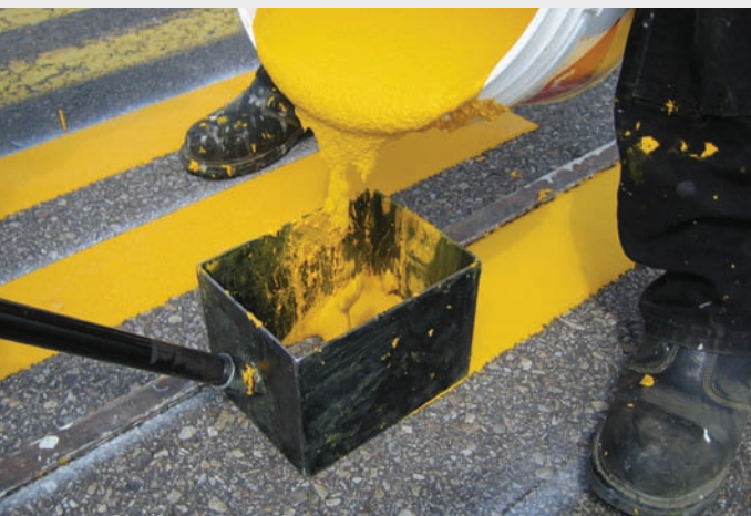
Transverse marking application
