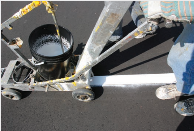
Cold Plastic applied using a walk-behind applicator
