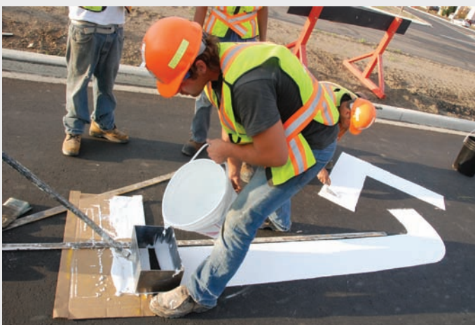
Message markings are applied using a draw box
